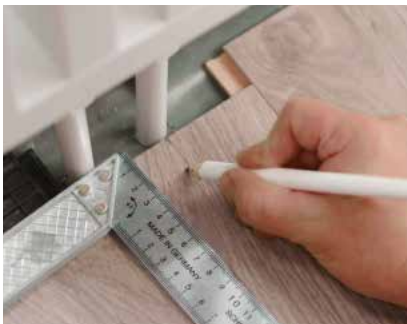
Door frame and radiator pipes
